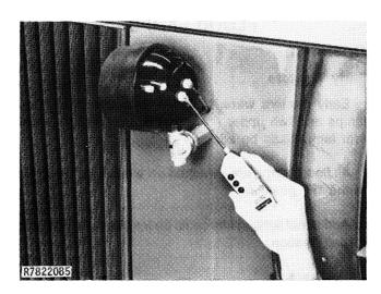
Fig. 8-Using Voltage Detector
