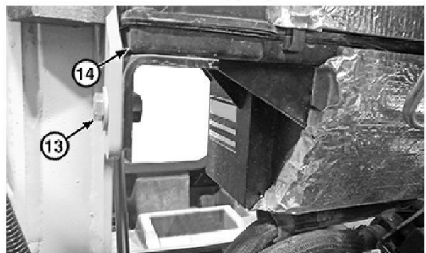
TX1255898A-UN: Air Conditioner and Heater (left side view)
